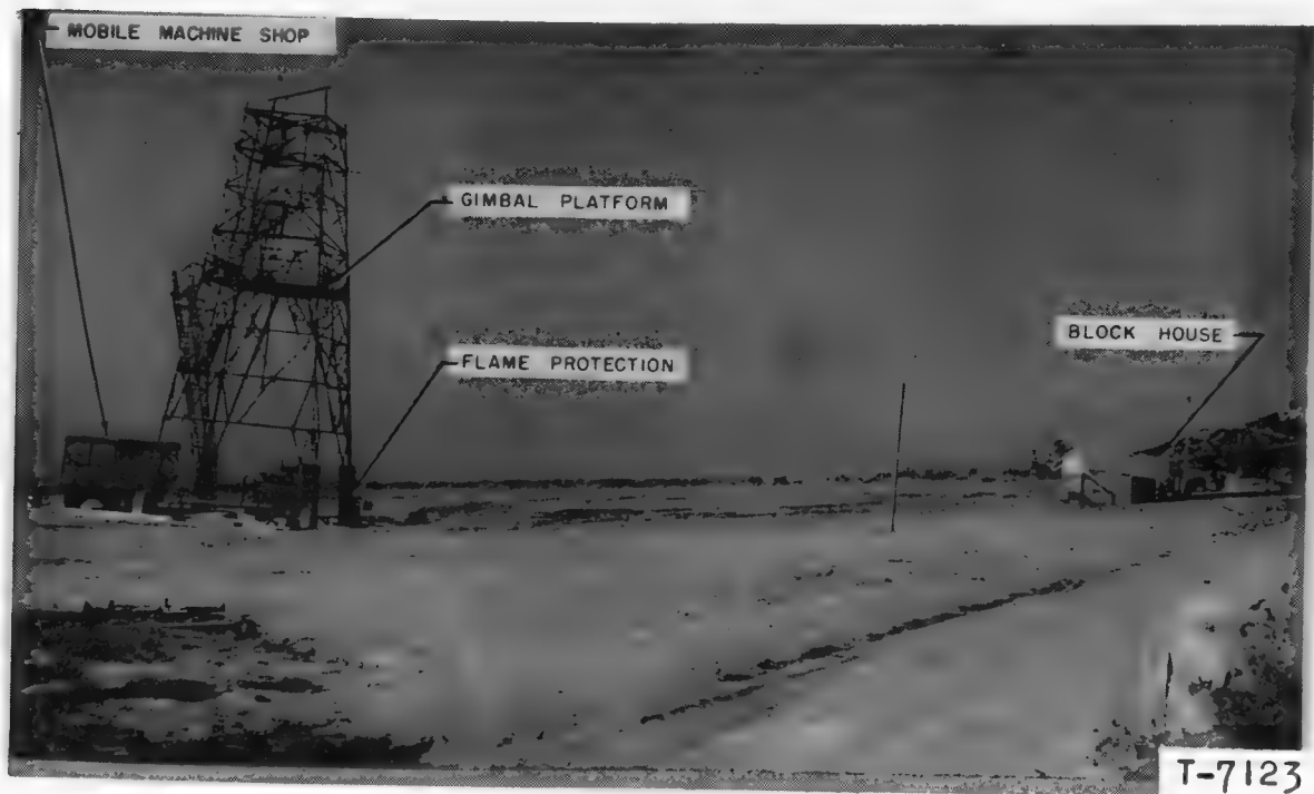
FIG 45 -- STATIC FIRING SITE AT POINT LOMA IN EARLY PREPARATION
